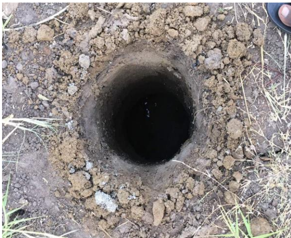
FOUNDATION PILE FOR SOLAR PANEL
