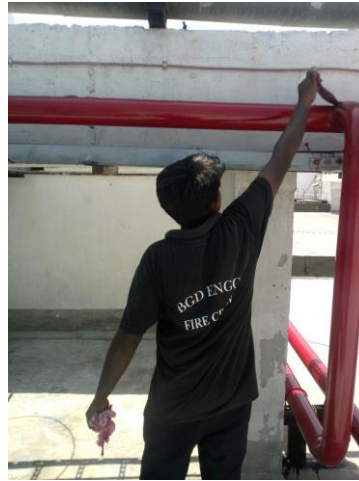
Fig 28 Fire fighting system fabrication and maintenance
