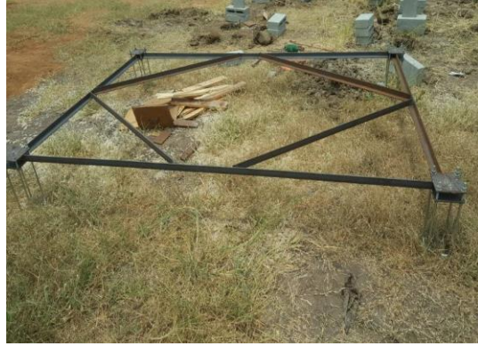
TEMPLATE FOR FIXING J BOLT IN FOUNDATION
